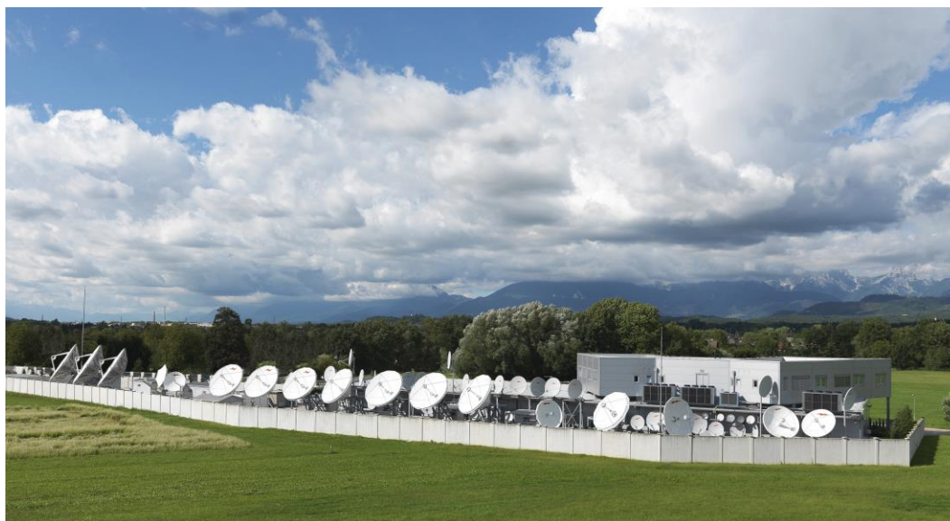
STN Facility Antenna, Slovenia, Image Courtesy STN
